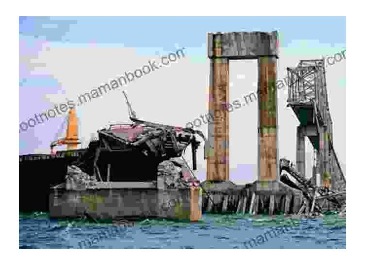
On May 9, 1980, a freighter ship collided with the Sunshine Skyway Bridge. The impact of the collision caused a section of the bridge to collapse. Thirty-five people were killed in the collapse.
